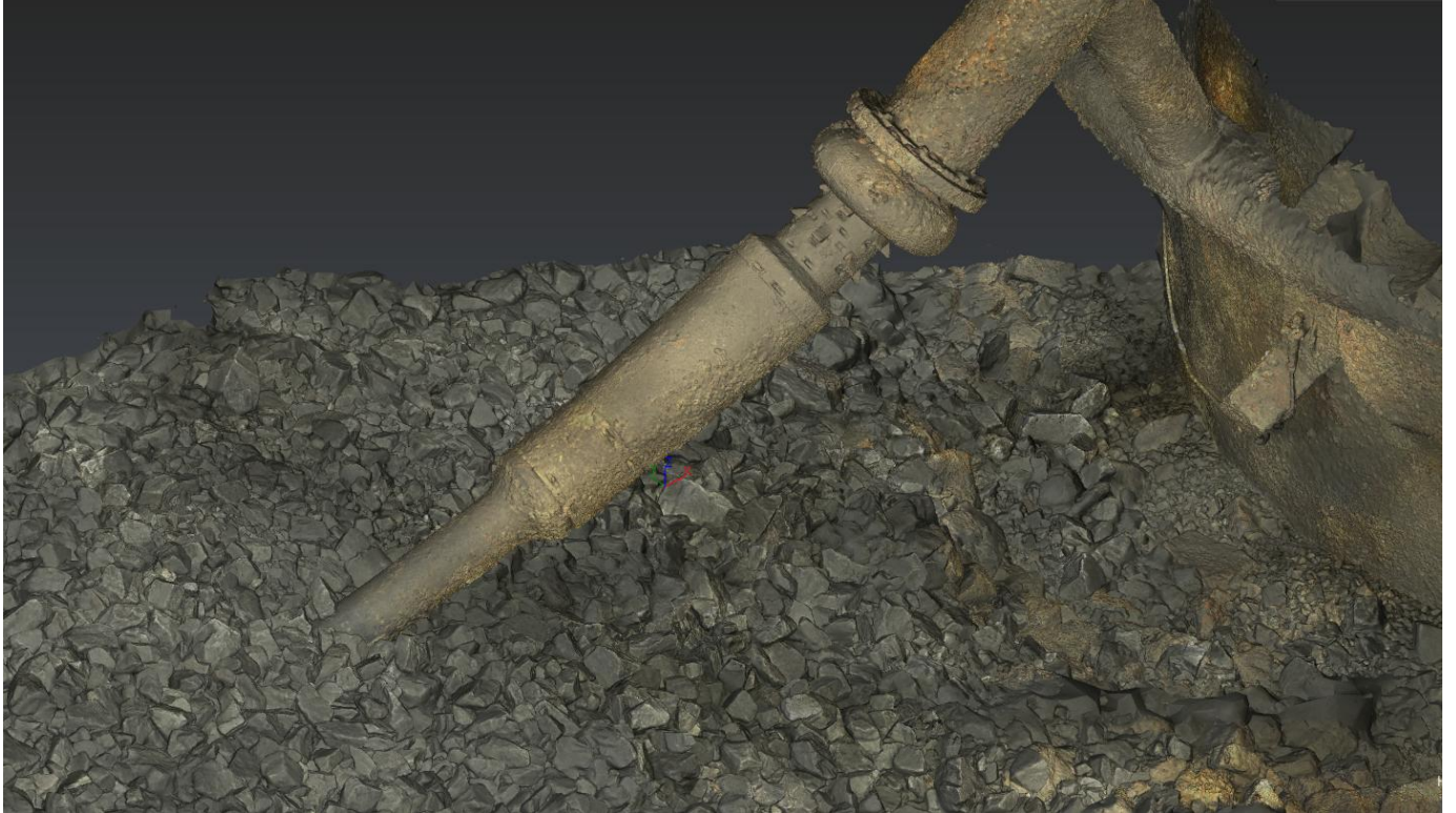
Image showing the Dense Cloud 3D model of the anomaly area on the OSP East CPS cable after the rock dump operations
